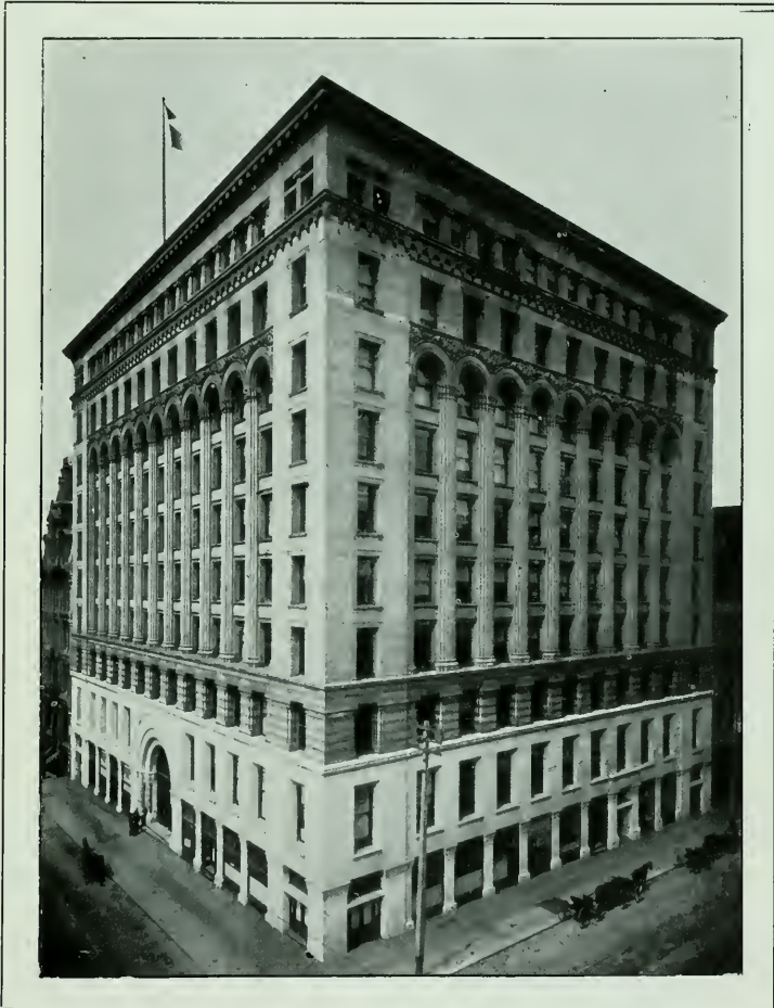
MILLS BUILDING. Cor. Montgomery and Bush Streets.
